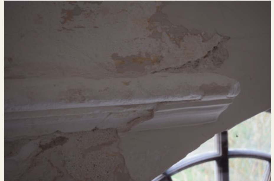
Detail of plaster cornice before restoration with damaged plaster removed.
